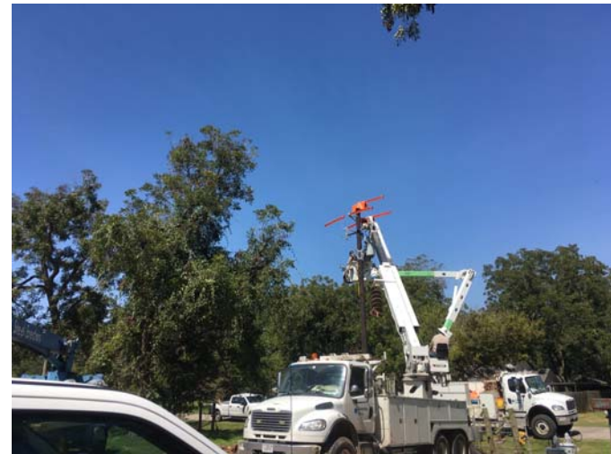
5. Installation of electrical provider service pole
