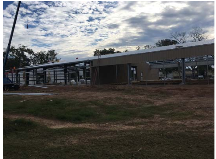
8. Installation of PEMB roof sheathing
