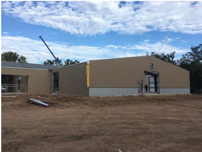
7. Installation of PEMP wall sheathing
