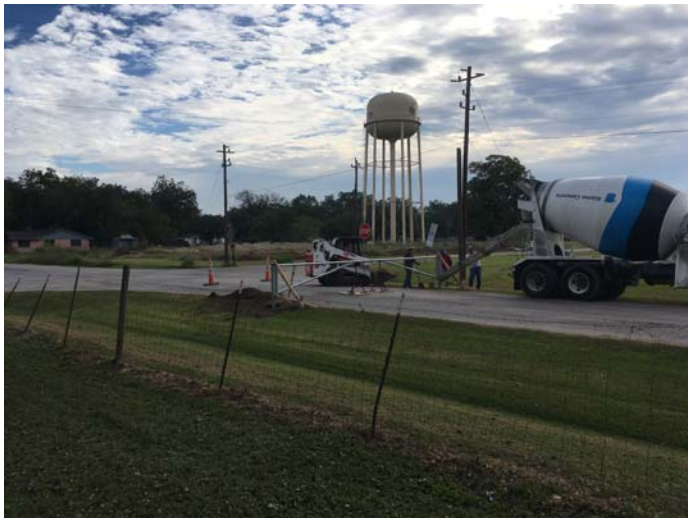
9. Installation of security gates at abandoned R.O.W.
